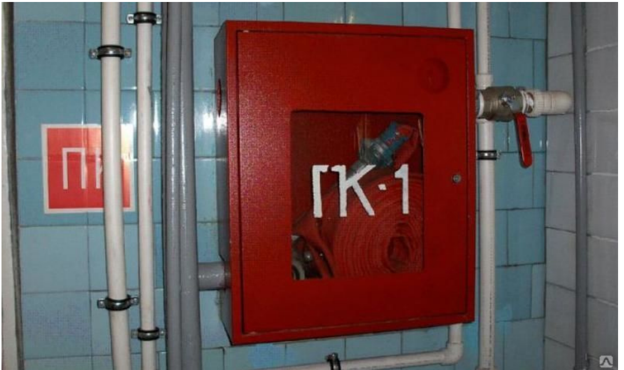
Figure 3. Fire cabinet with ligature ПК in the city of Perm
